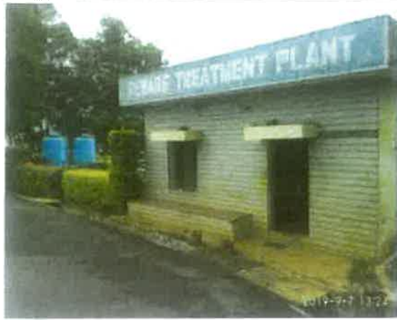
Fig. 4 Sewage Treatment Plant
